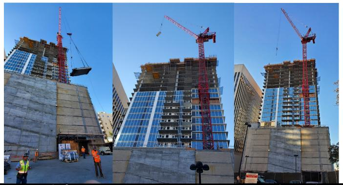
"By using RediStair®, we were able to have stair access one floor behind our wet deck for over 40 floors. No extra ladders, no scaffold stairs. The threaded inserts in the handrail embeds made installing temporary rails fast and easy with no additional touch up. I will be looking at using RediStair® as a CIP solution on any future projects that I can."
